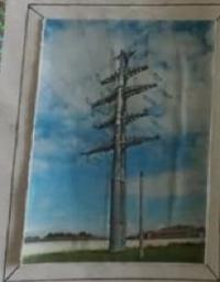
The load bearing capacity is more in steel tubular pole in comparison to wooden pole and concrete pole. But due to excessive cost. These poles are used for 11KV/33KV volt low and medium current system. In some cases for use poles high volt in 33 KV.
